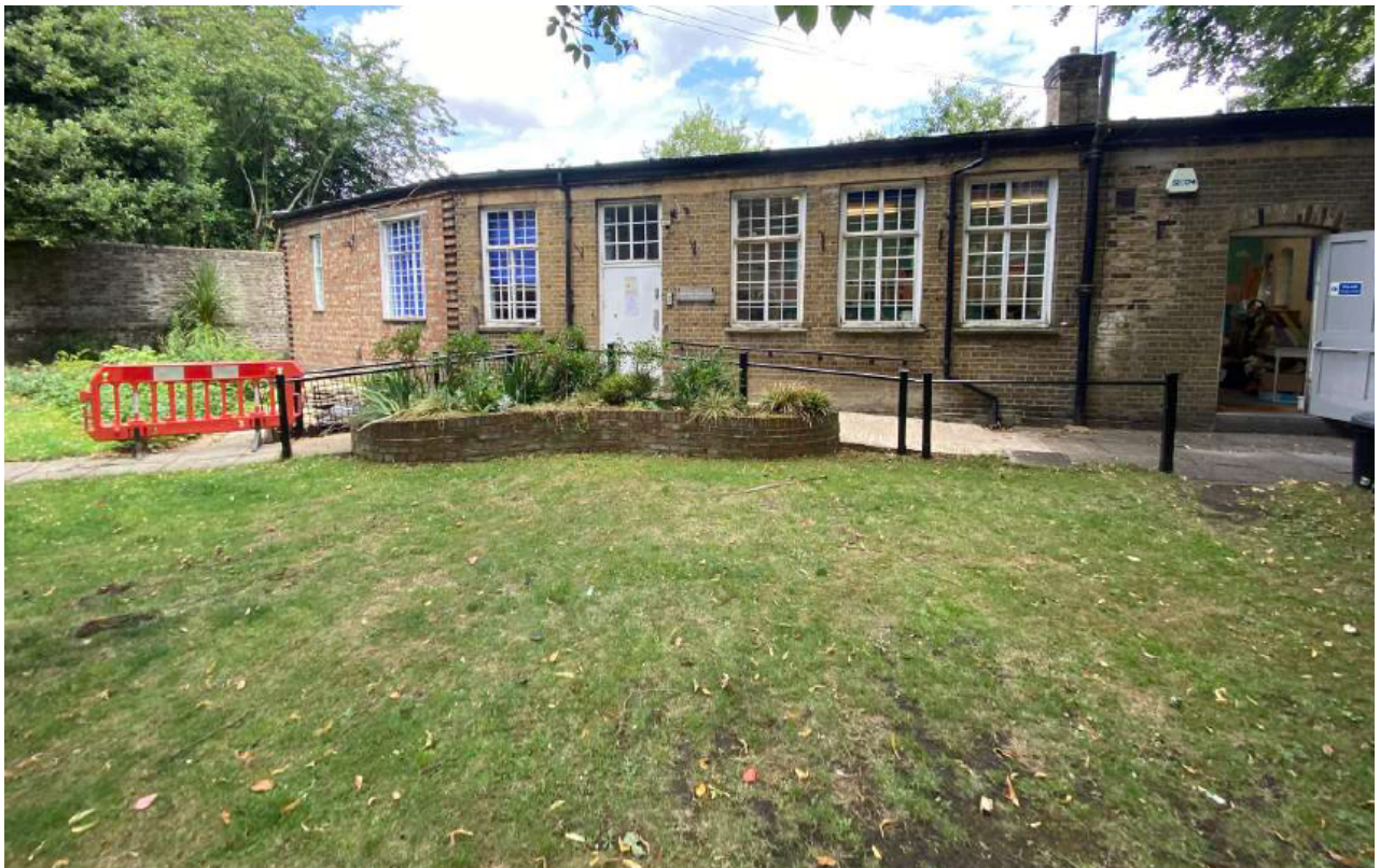
Image 5: Front elevation of Dame Geraldine Hall
