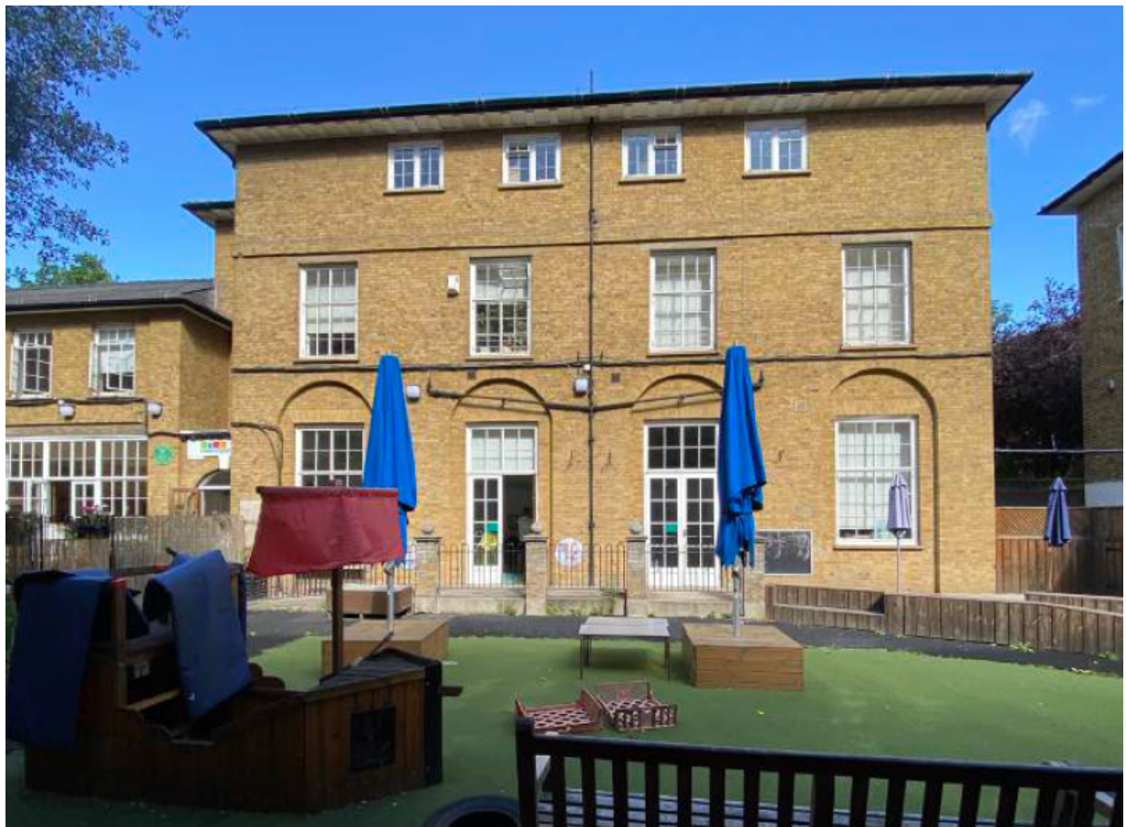
Image 3: Front elevation of No. 6-9 Manor Gardens (containing No. 7 at ground floor)
